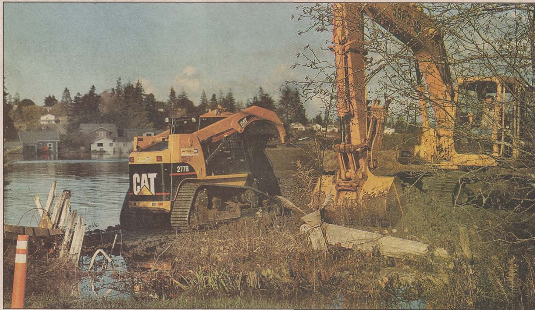
World Photo by Susan Chambers Heavy equipment operators go to work building a gravel road out to the dike in Libby that broke on Friday. Several dump trucks hauled rock to build the road. The houses in the background, on Old Wireless Lane, have been flooded since Friday.
